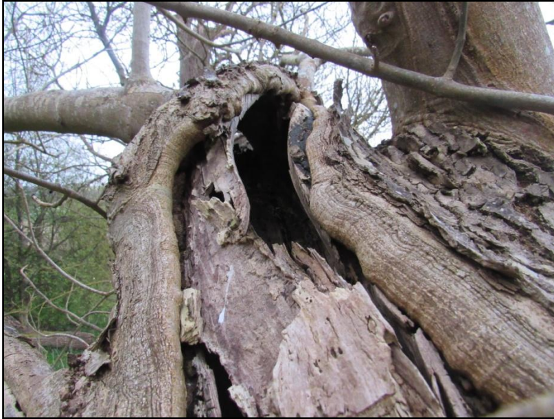
Figure 16. The main stem has been badly damaged by fire and is now completely hollowed out leading to numerous hollow branches. All of these locations were thoroughly inspected and there was no evidence to indicate the presence of birds or bats.
